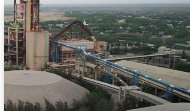
3. Conveying Belts 315 m
