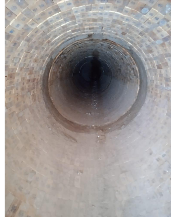
New Refractory installation for 65 M
