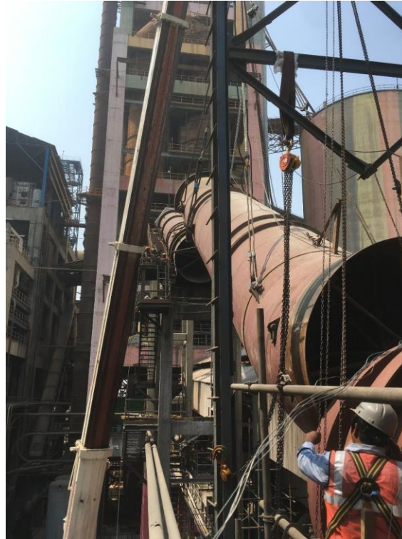
TAD Duct replacement 45 M
